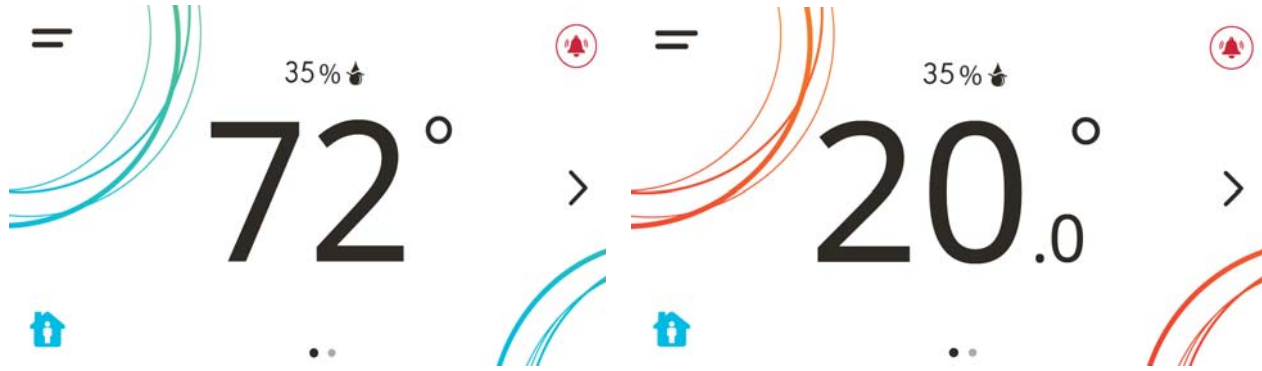
Figure 17: Thermostat controller home screen in cooling mode (left) and heating mode (right)
